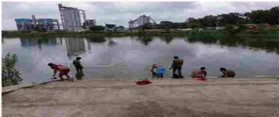
Pond renovation near surrounding village area by DCBL Bokaro to conserve the rain water
