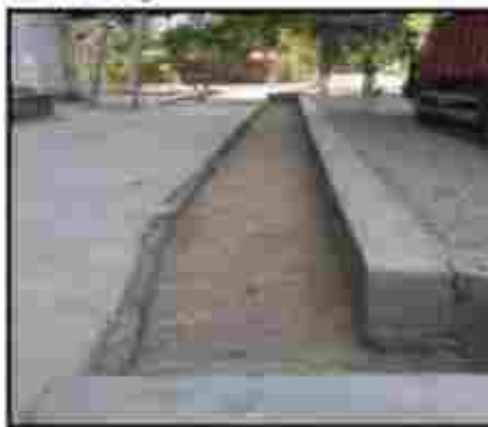
Rainwater harvesting/recharge trench near bag house and near cement mill 2 area
