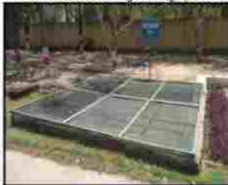
Rain water harvesting recharge pit near FHG Hostel & Rain water recharge trench in-front of CCR main building
