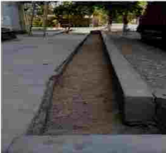
Rainwater harvesting recharge trench near bag house and near cement mill 2 area
