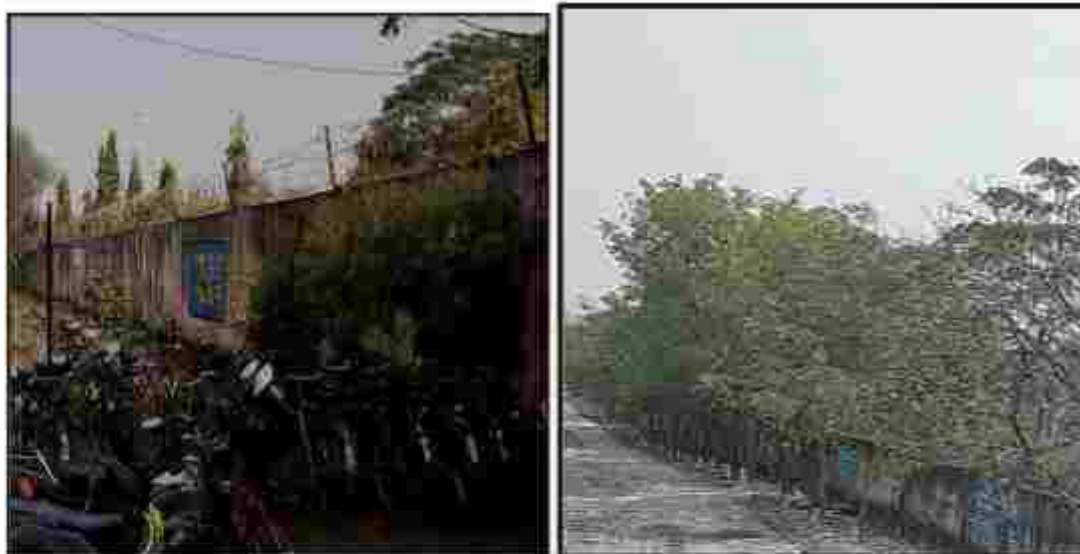
Boundary wall constructed in around the plant
