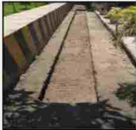
Rainwater harvesting recharge trench near CCR building 3 near E type quarter
