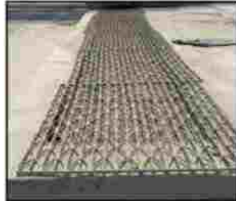
Rainwater harvesting/recharge trench near bag house and near cement mill 2 area
