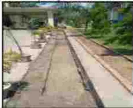
Rain water harvesting recharge pit near FHG Hostel & Rain water recharge trench in-front of CCR main building
